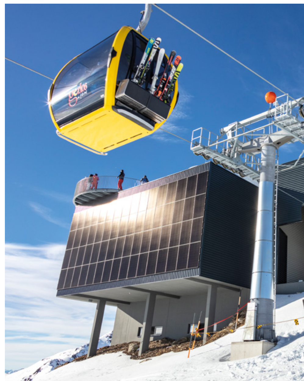
The Stuanmandlbahn in Gerlos features the latest addition to Zillertal Arena's eight PV systems.
