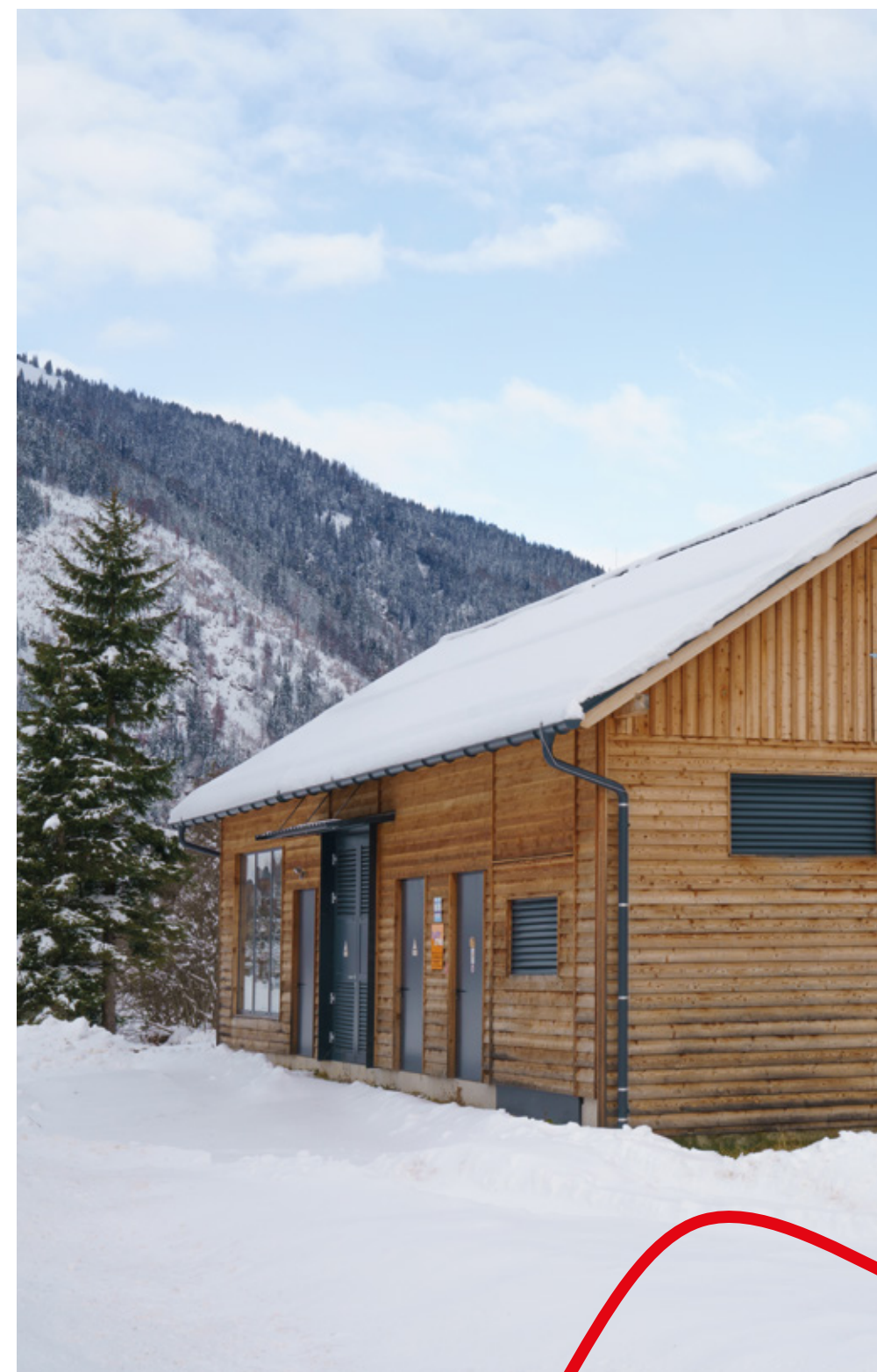
The snowmaking power plant seamlessly blends into Riesneralm's valley station.
